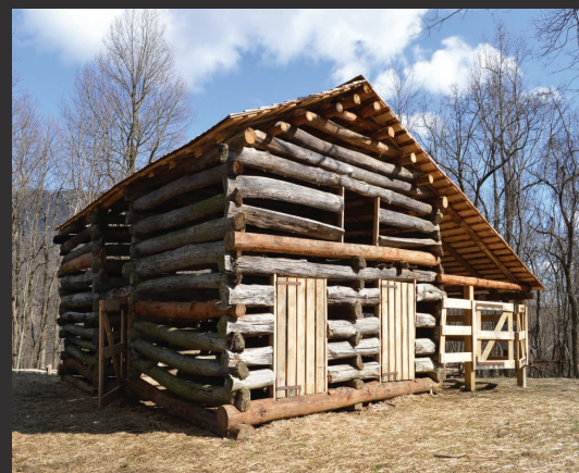
The barn at Johnson Farm after repairs
