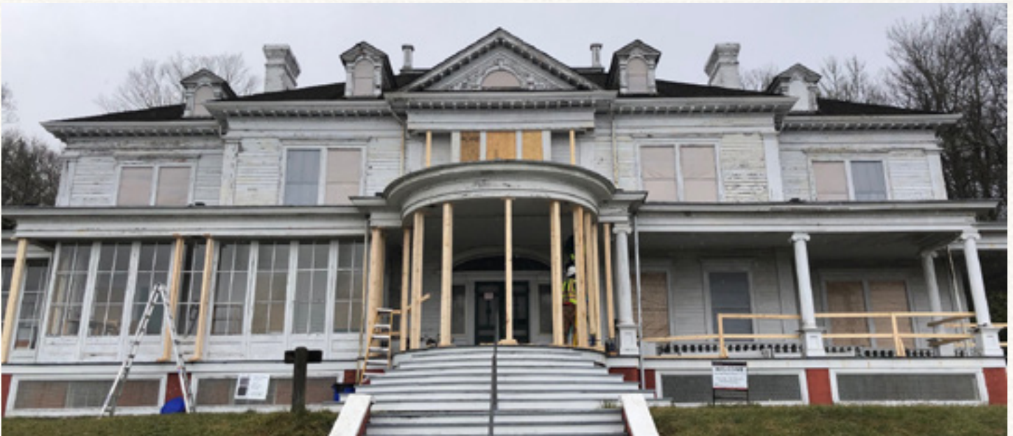
Above: The manor with windows & railings removed.
