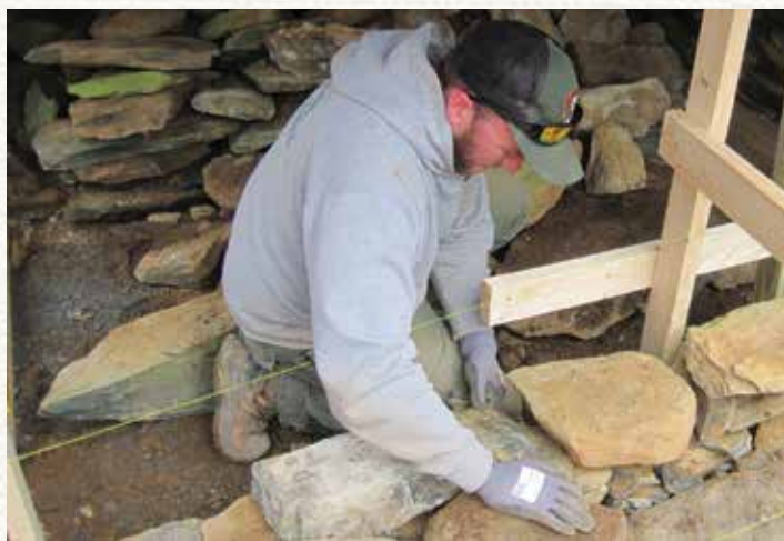
Historic Preservation Training Center specialist Issac Foreman demonstrates the proper way to stack and lock dry stones.
